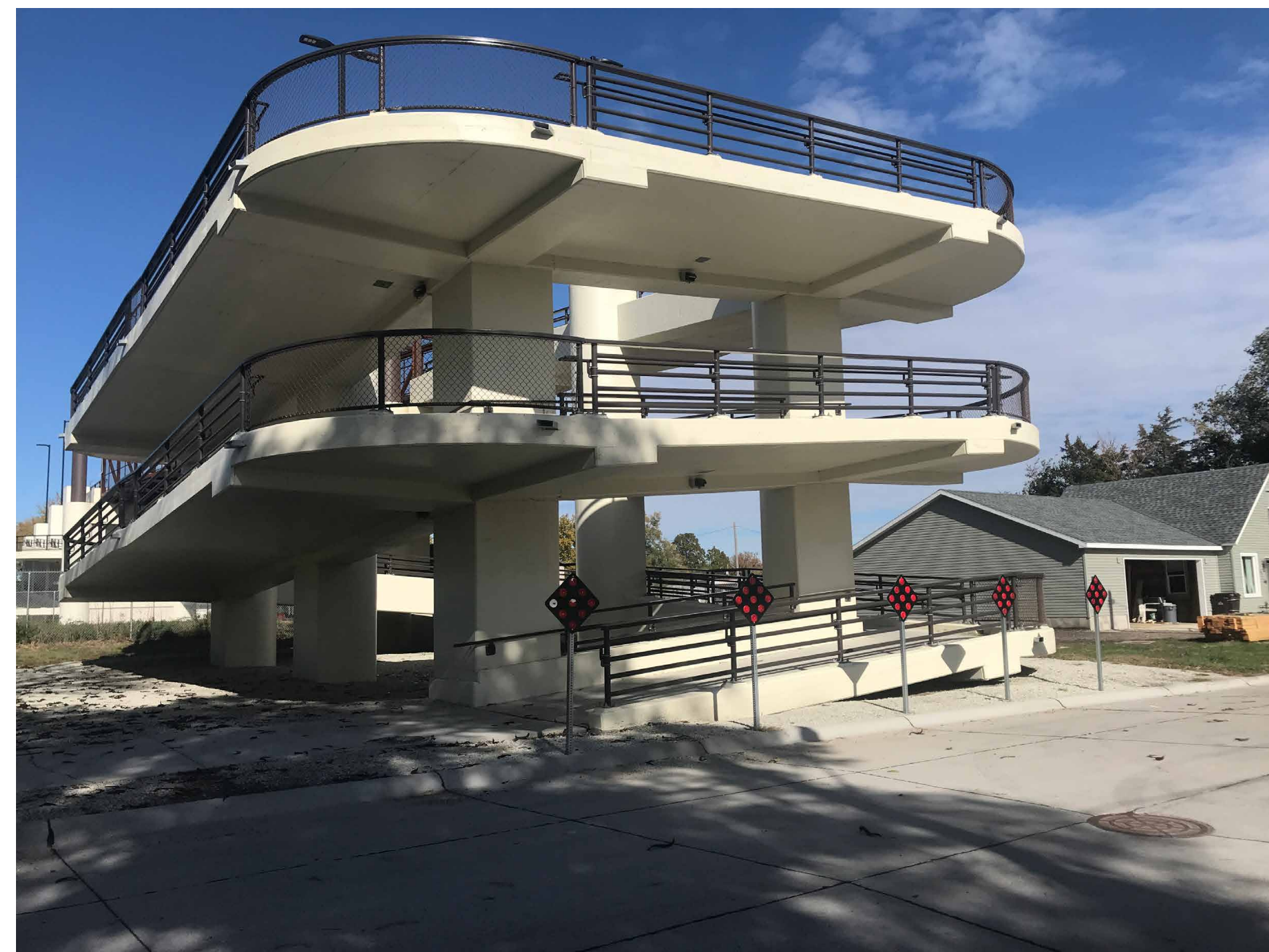
18th Street Pedestrian Bridge.
