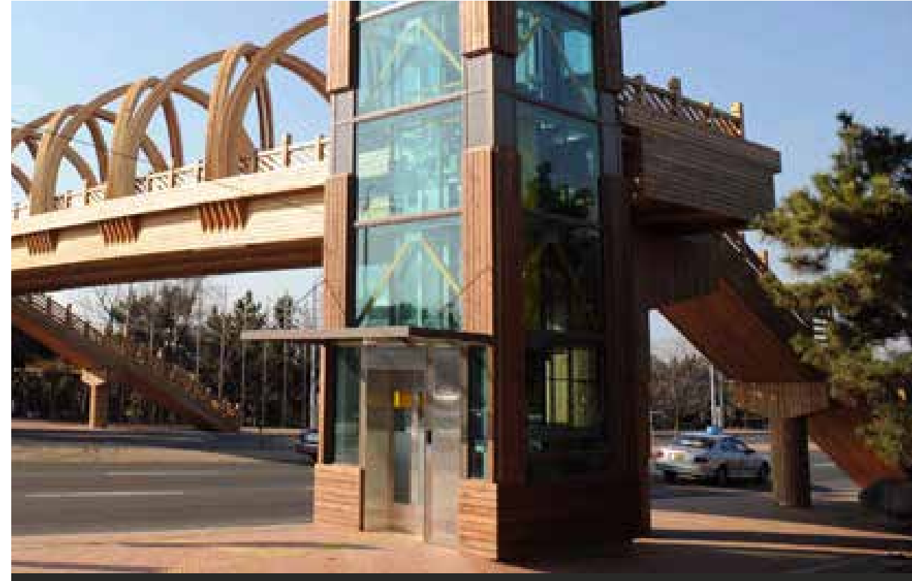
Elevator and stairs to overpass.
