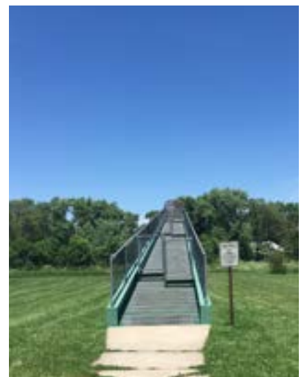
Existing Pedestrian Bridge
