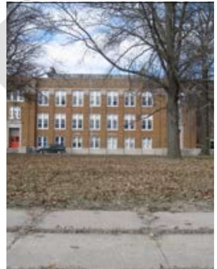
Reuse / Redevelopment Opportunity
