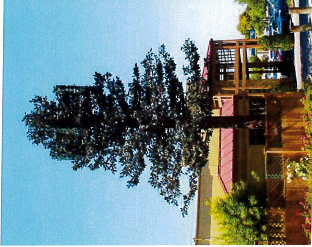
45' Monoelm 2.6 branches/ft Full cladding
