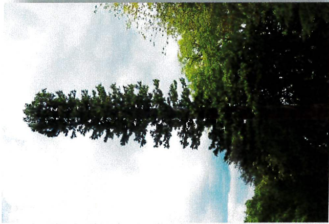
100' Monopine 2.6 branches/ft Standard cladding
