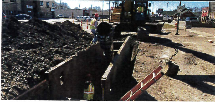
Exhibit A: Lincoln Avenue Water Main replacement
