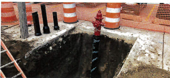
Exhibit B: Lincoln Avenue Water Main replacement
