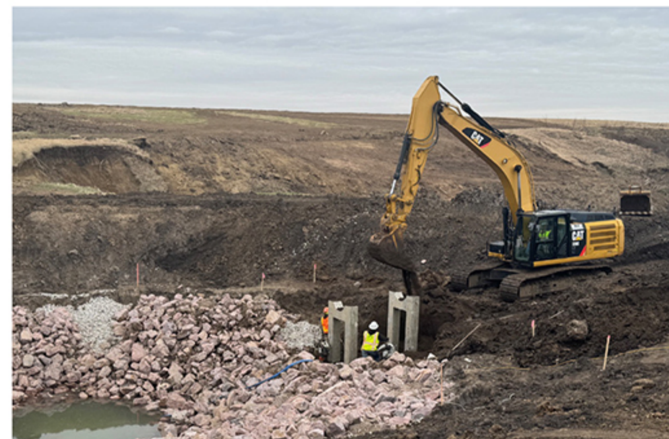
The plunge pool spillway outlet for site 27.
