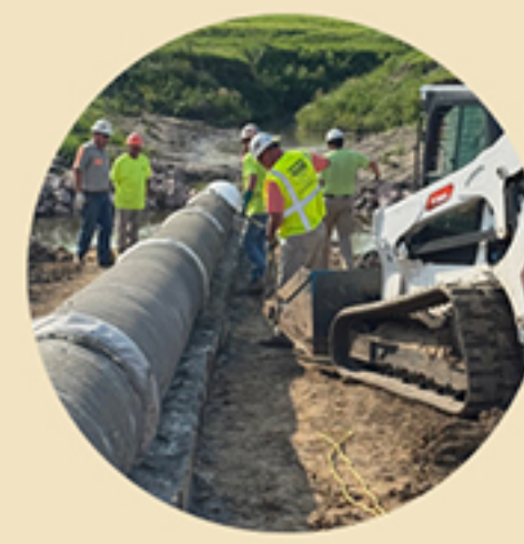
Wahoo Creek Watershed Construction Page 3
