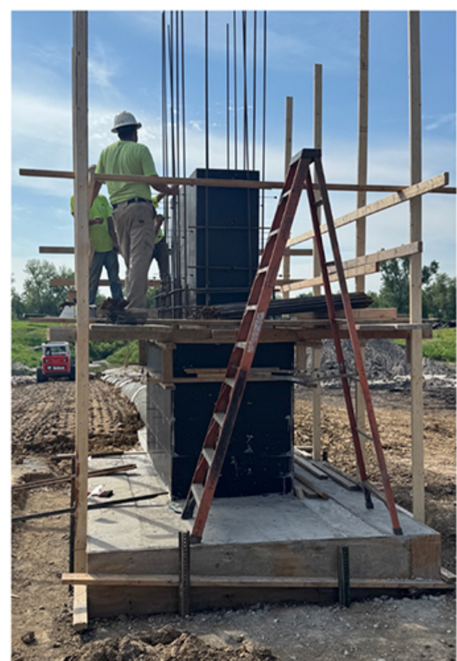
The riser inlet under construction at site 27.
