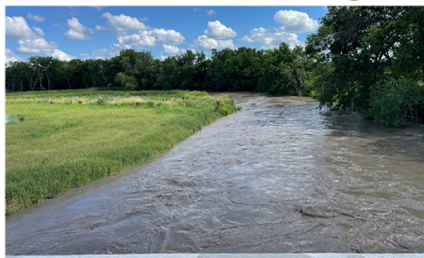
The "final bend" benching project looking south from the new county road bridge after recent heavy rains that historically would've caused localized flooding but were contained within the Shell Creek banks.
