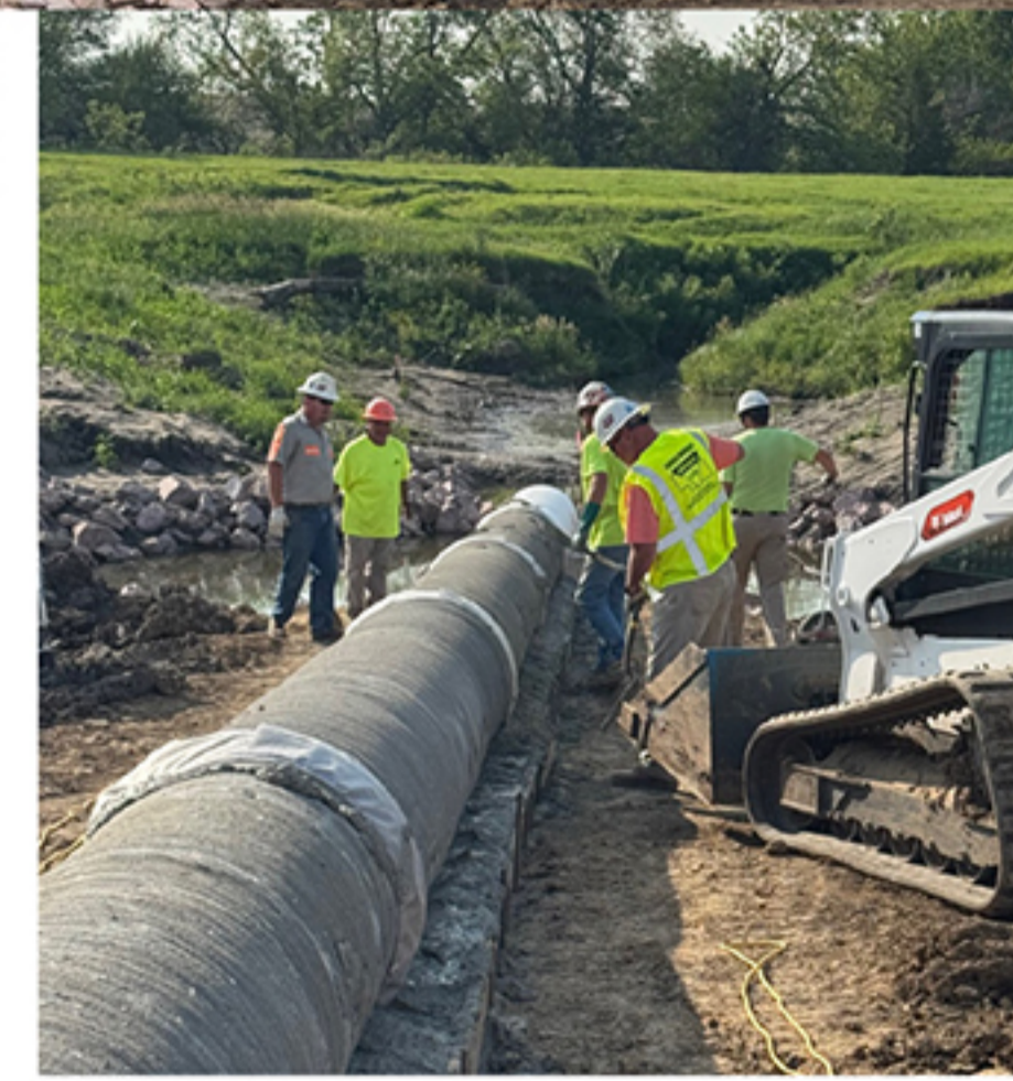
Workers grouting the 24" concrete pipe spillway.
