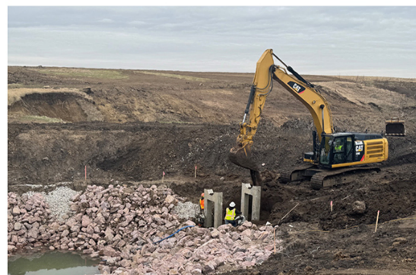
The plunge pool spillway outlet for site 27.
