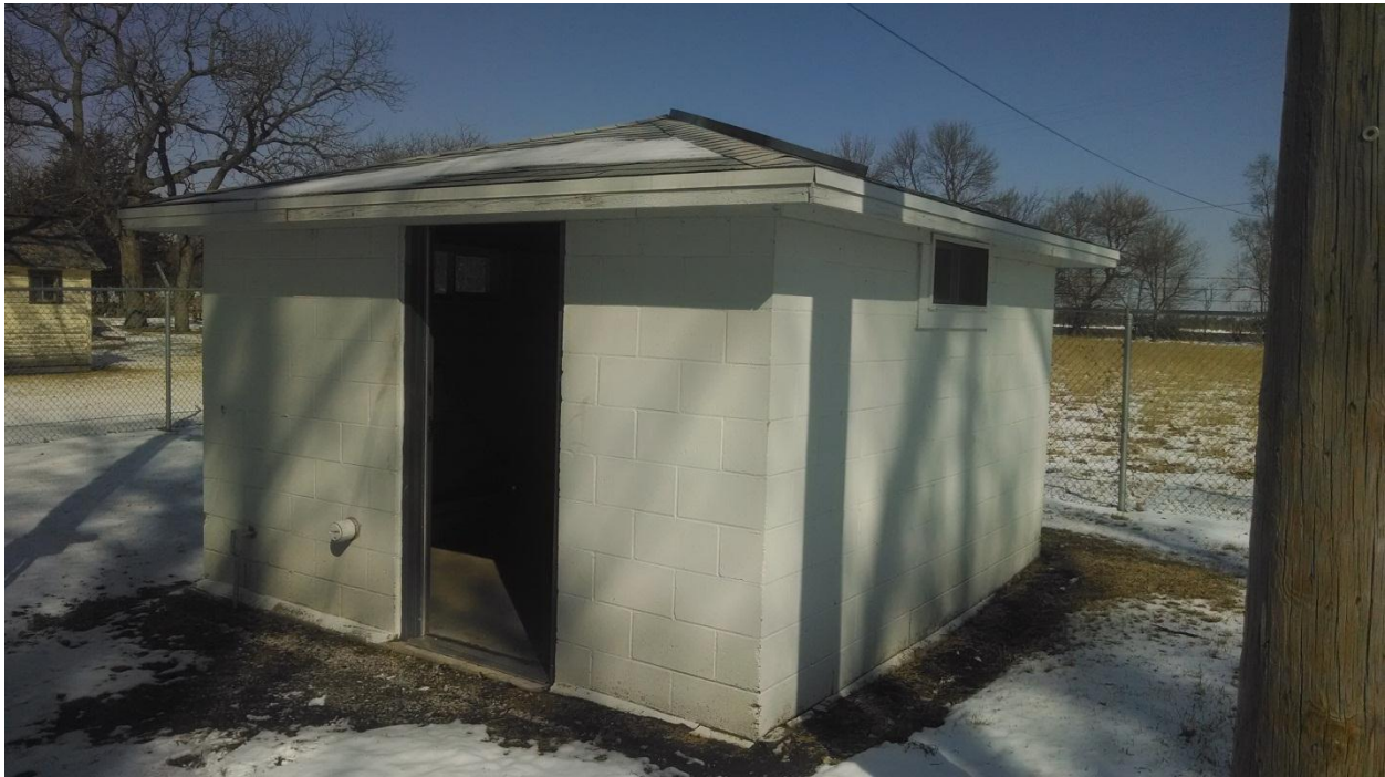
Figure 2-8: Well 71-1 (East Well)
