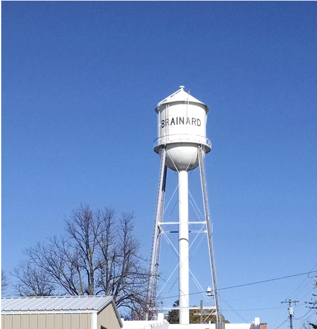
Figure 2-16: Brainard's Elevated Storage Tank
