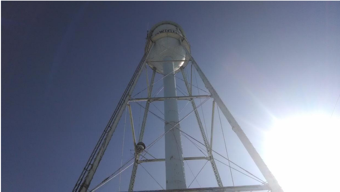
Figure 2-17: Dwight's Elevated Storage Tank
