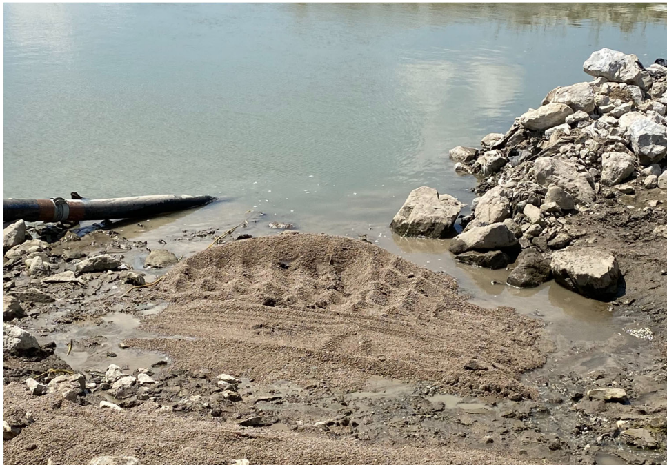
Photo 6 – Aggregate/Rock being used to cover discovered boil
