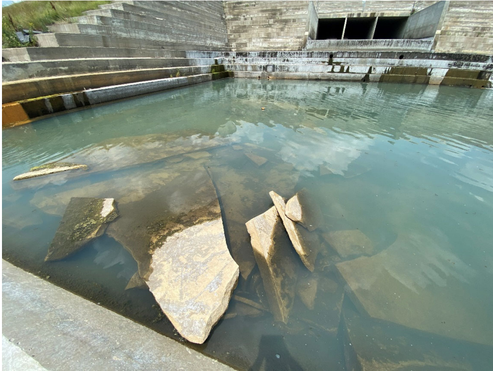
3 – Spillway apron surfacing piled up
