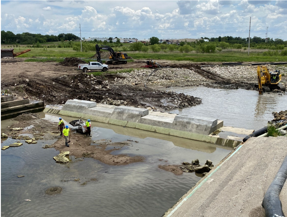
1 – View of contractor cleaning debris from basin
