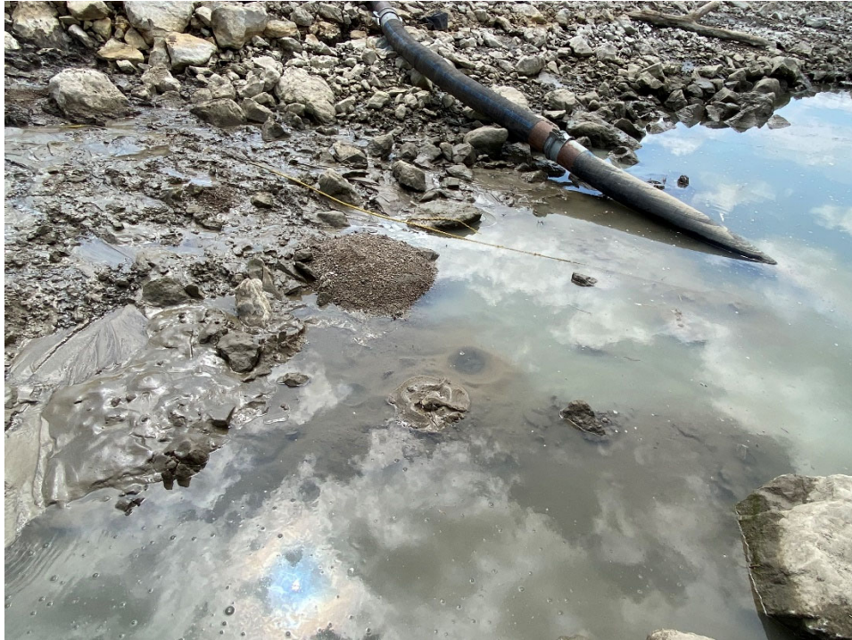
Photo 5 – Micro boil appearing along water's edge in stilling basin
