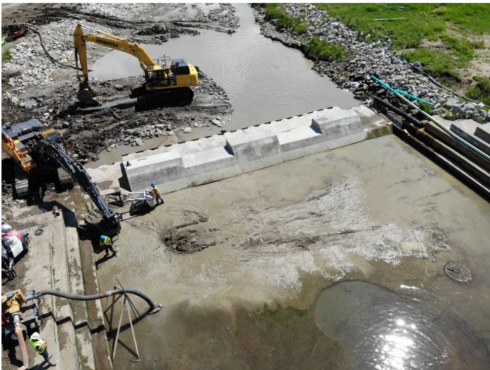
2 – Aerial view of stilling basin
