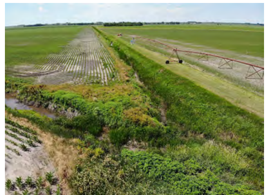
The confluence of the NBCD and the O'Hare ditch shows how inefficient hydraulics can cause sediment deposition.
