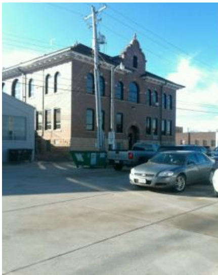
Power company transformers ↑
