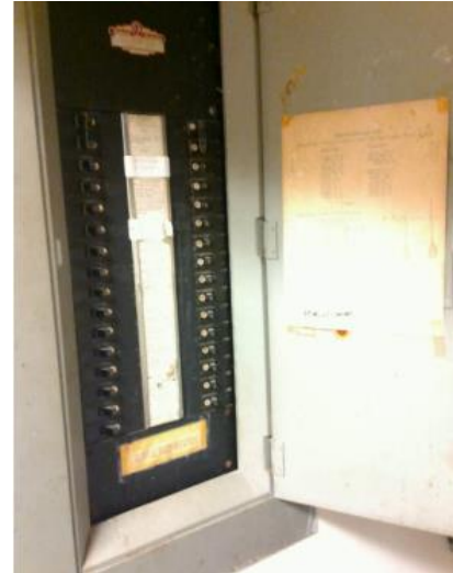
First floor panel ↑
