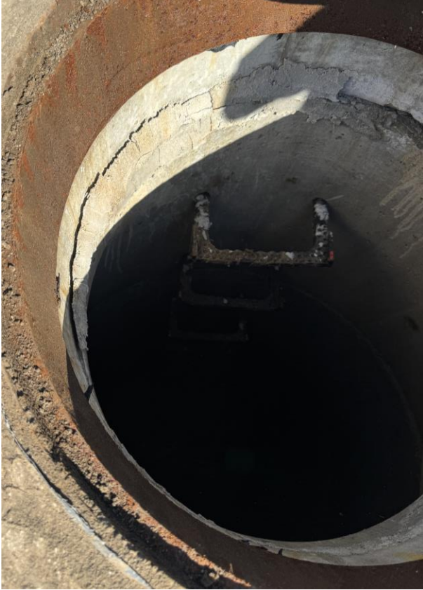
Photo 1: grout in manhole
