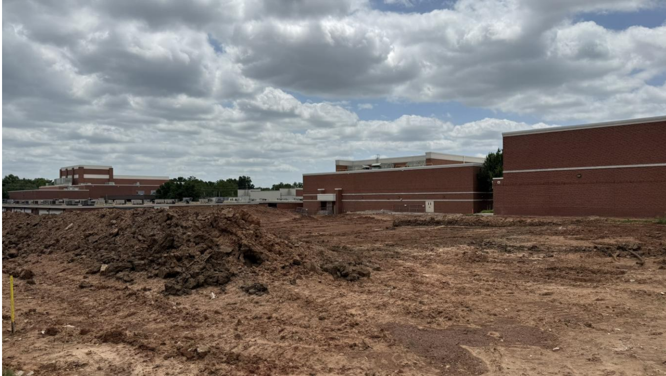
DEMOLISHED WEST GYM AND CITY GYM BUILDINGS
