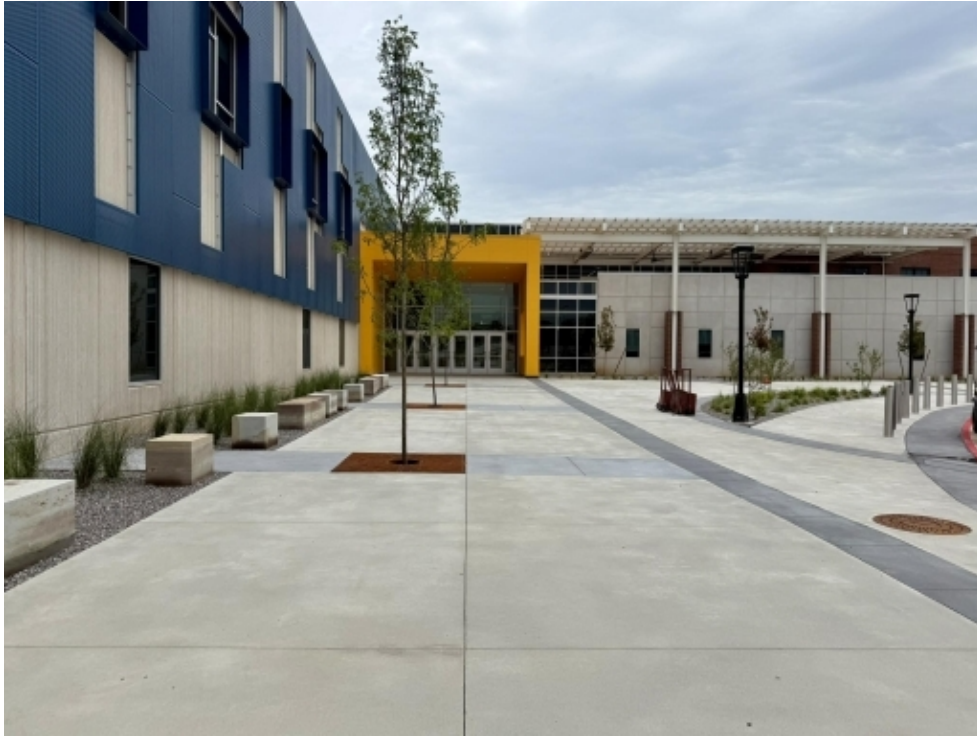
FRONT ENTRY AND DROP-OFF
