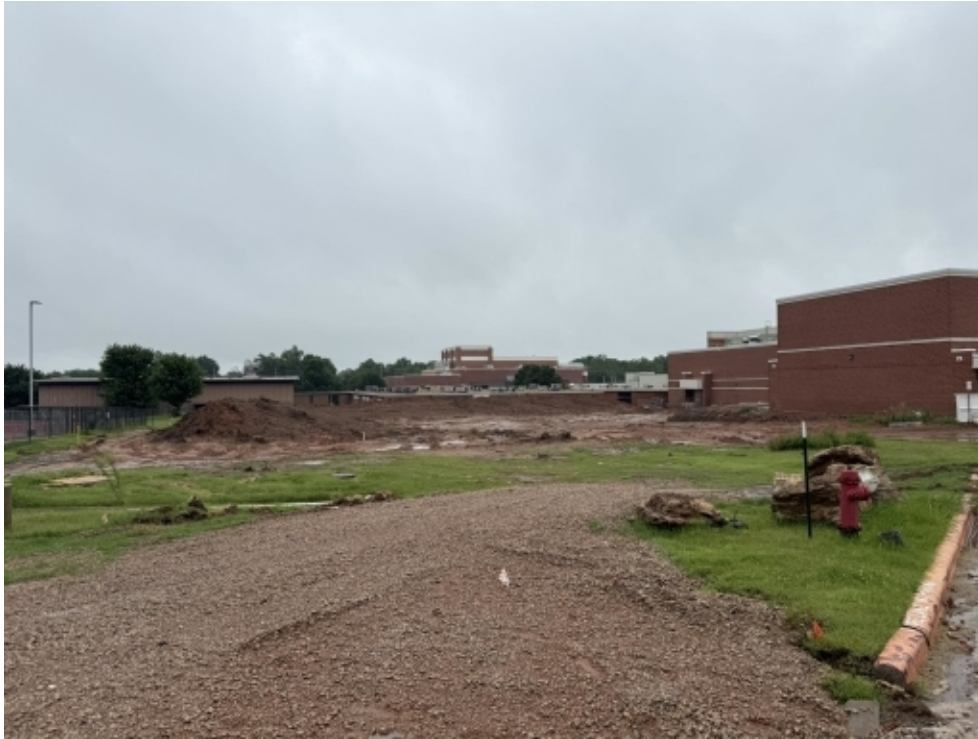
DEMOLISHED WEST GYM AND CITY GYM BUILDINGS
